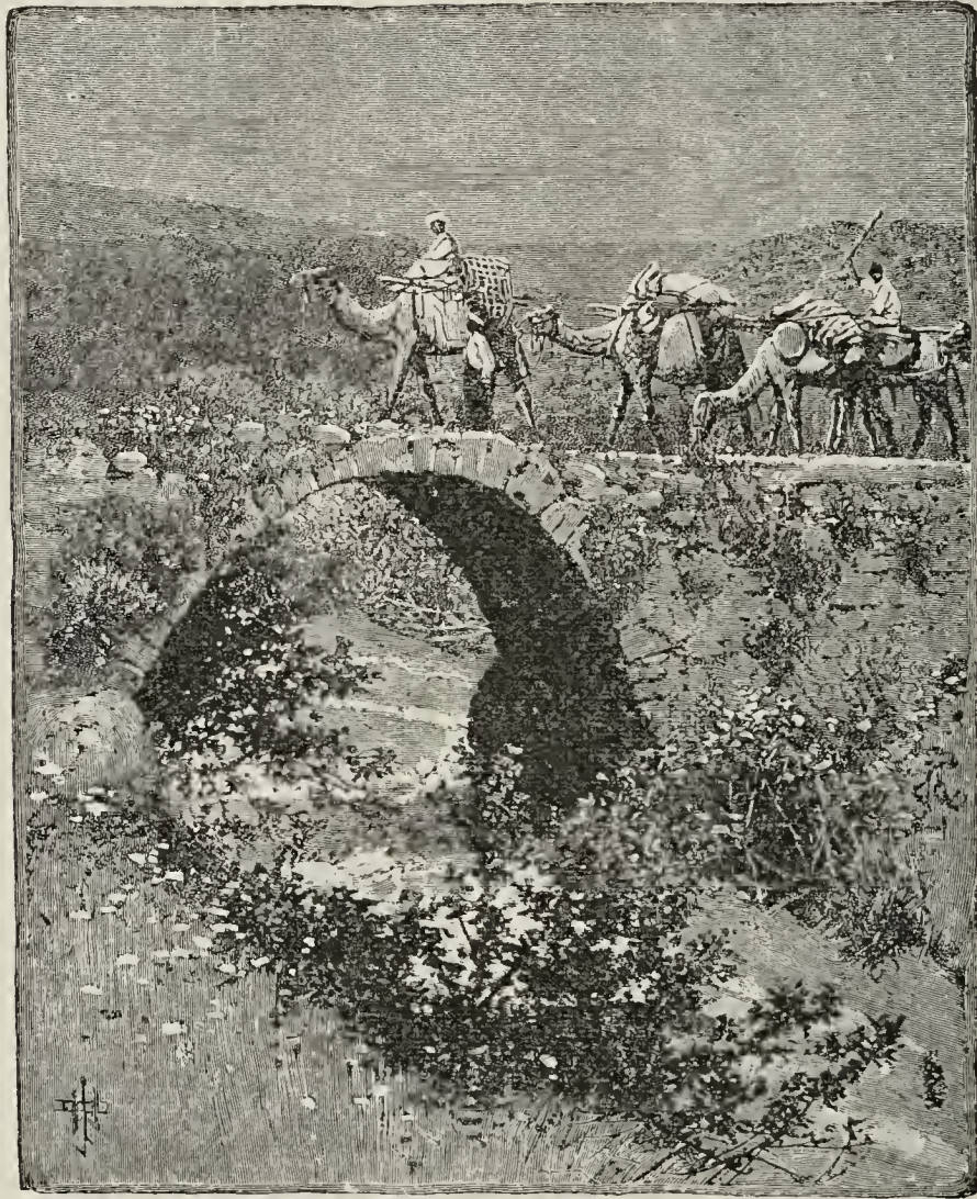
Bridge over the Hasbany.
